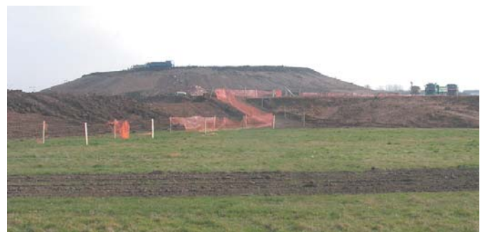
Above: View looking east towards Mound 3 from the western park boundary.
